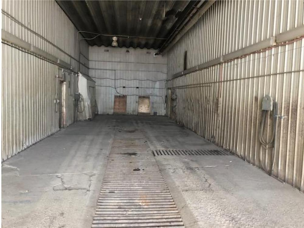
**FIGURE 17 – SHOP BAY WITH DRAINAGE SUMP**
