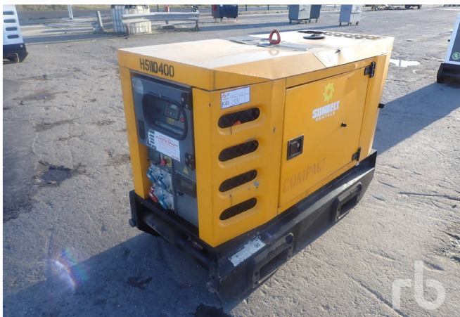
2016 SDMO R22 SKID MOUNTED
