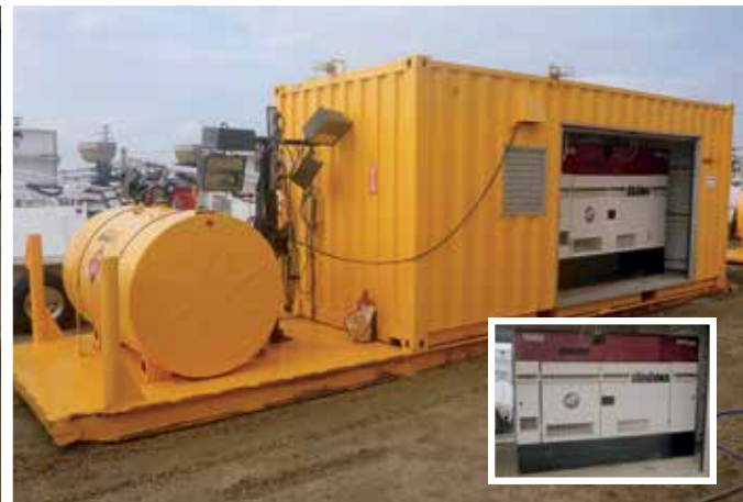
1 of 6 – Enclosed 2013 Shindaiwa 100 KW
